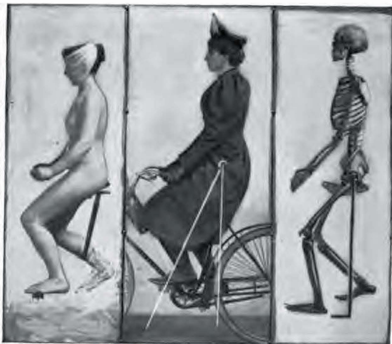
FIG. 3.—The rider well over her work, the foot forward at the point where most of the power is applied, showing how short a distance from the perpendicular the pedal sweeps forward. Illustrating a low position of the handle bars, with an arm that is too straight.
