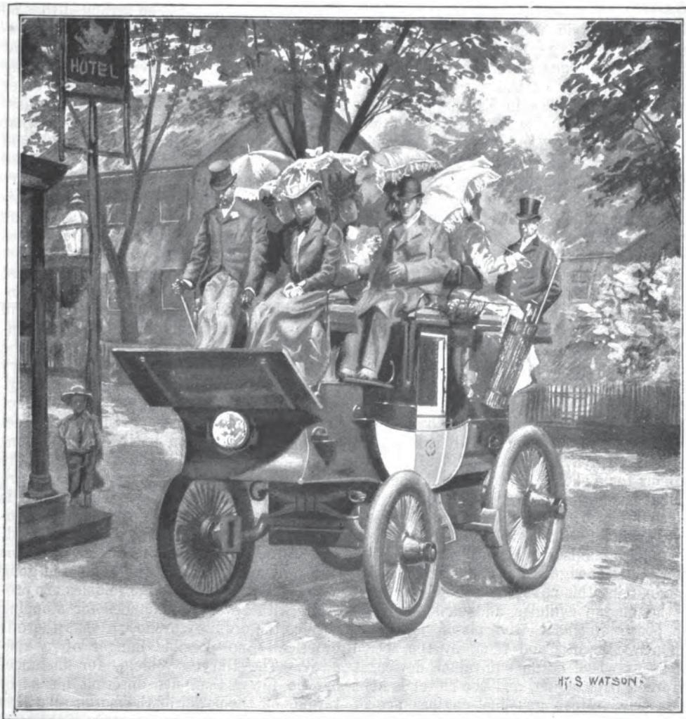
A MOTOR TALLY-HO, PROPELLED BY STORED ELECTRICITY.
